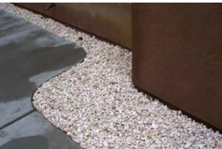
Figure 1. The best type of foundation landscaping.
